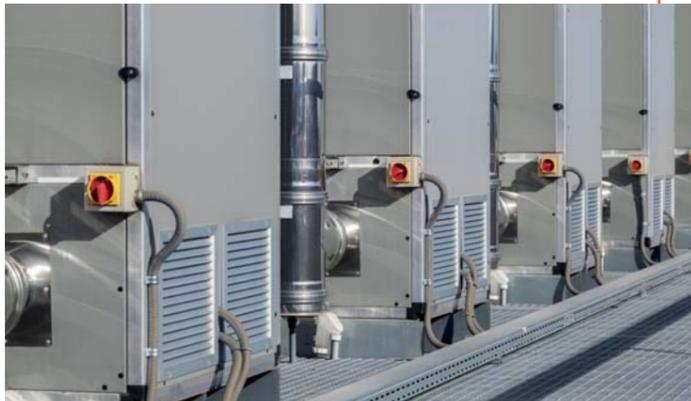
Replacement of obsolete compressors with new, more efficient models allows for the production of the necessary compressed air with significantly less electricity. The wasted energy, which is shed via heat during the compression process, can be recaptured and used for other purposes with the right heat recovery equipment.
