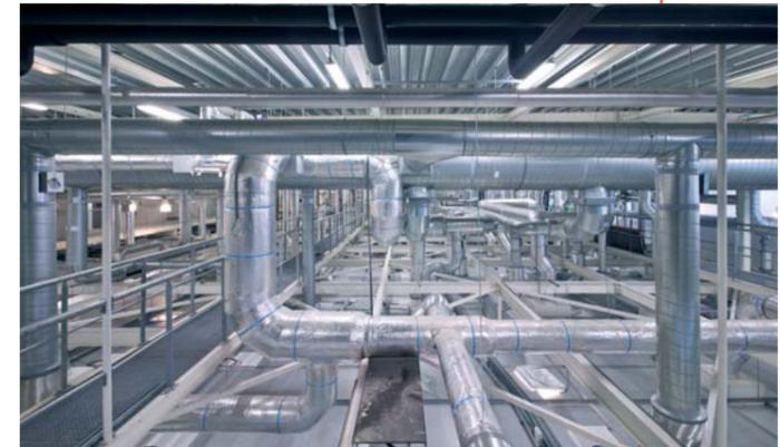
Leaks, incorrect duct dimensions, and ductwork systems that have been gradually expanded or modified over many years can lead to a very energy-intensive air movement process in order to get the conditioned air to the spaces where it is actually needed within the facility. The optimization of the ductwork and other air distribution channels always has a positive effect on the operation of ventilation equipment across the entire system.
