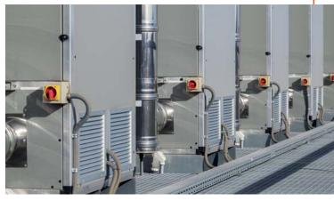
Replacement of obsolete compressors with new, more efficient models allows for the production of the necessary compressed air with significantly less electricity.
