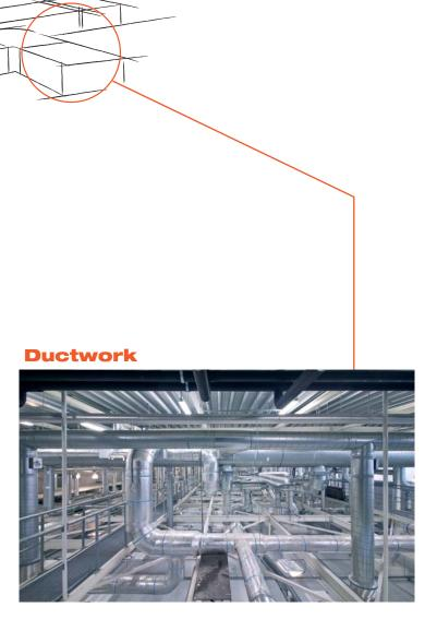
Leaks, incorrect duct dimensions, and ductwork systems that have been gradually expanded or modified over many years can lead to a very energy-intensive air movement process in order to get the conditioned air to the spaces where it is actually needed within the facility. The optimization of the ductwork and other air distribution channels always has a positive effect on the operation of ventilation equipment across the entire system.
